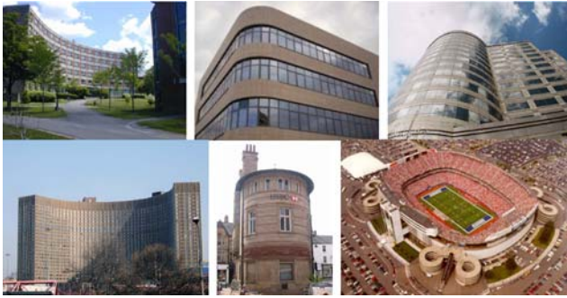
Fig. 3 Examples of non-conventional buildings of which the outer walls can be modeled as ruled surfaces, which have more flexibility than piecewise planar approximations
